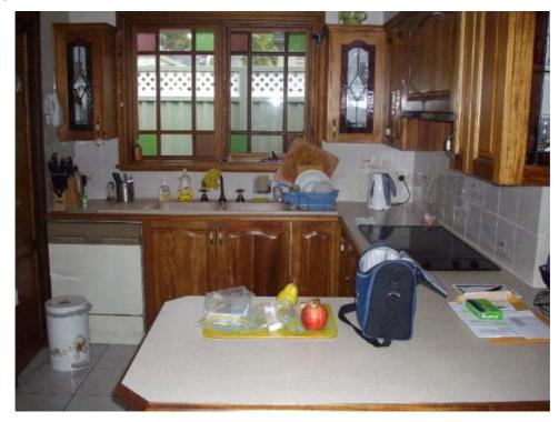
The kitchen cupboards are particle board with timber doors and laminated bench tops
